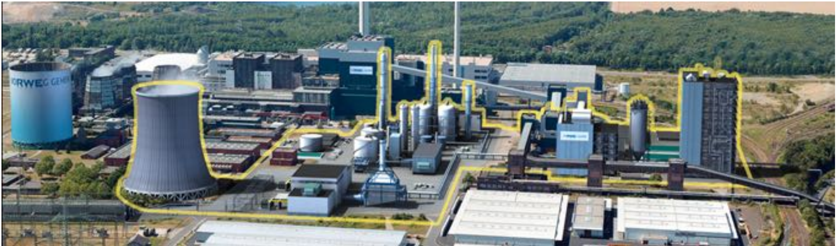
RWE IGCC power project (Source RWE website).
